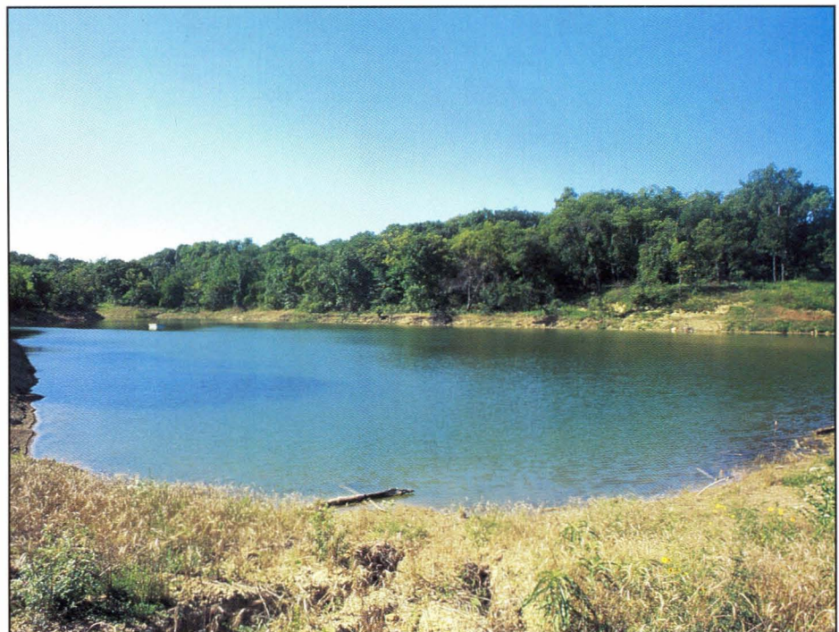
A view of the pond after the enormous job of enlarging the dam was complete. The family chose a contractor carefully, ensuring that the work was done with integrity.
