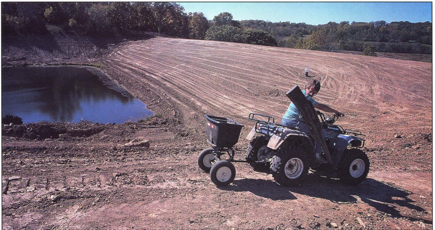
Mark Warnick plants wheat on the newly constructed pond dam to prevent erosion. The family also planted more than 1,000 trees, wildflowers, native grasses and forbs, as well as grain food plots. The efforts quickly paid off with increased wildlife sightings.
